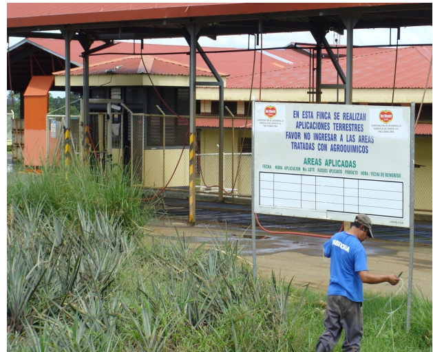
Photo 1. Agrochemical Storage facility. Babilonia Farm. Siquirres, Limon.
